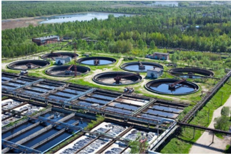
Settlement ponds are an effective part of the wastewater treatment process. (Credit: antikainen / iStock-Thinkstock)
