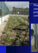
Plants are growing on roughly 30 cubic yards of recycled expanded polystyrene, and 5 cubic yards of composted organics and mulch.
